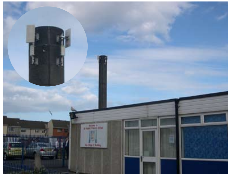
Base station deployment at primary school
