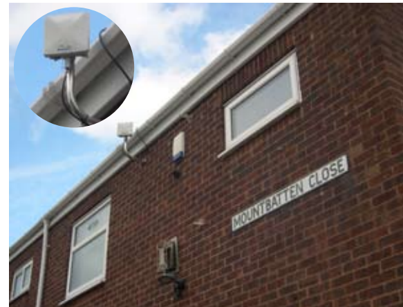
Antenna installation at one of the homes in Hartlepool
