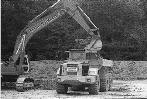
Removing the overburden
